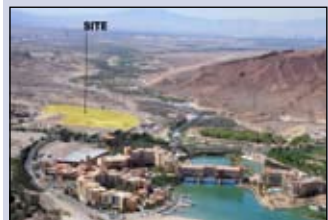
GALILEO PROJECT NORTH SHORE IN LAKE LAS VEGAS HENDERSON, NV 89011 23 ACRES $29,900,000.00 NICK TILL
